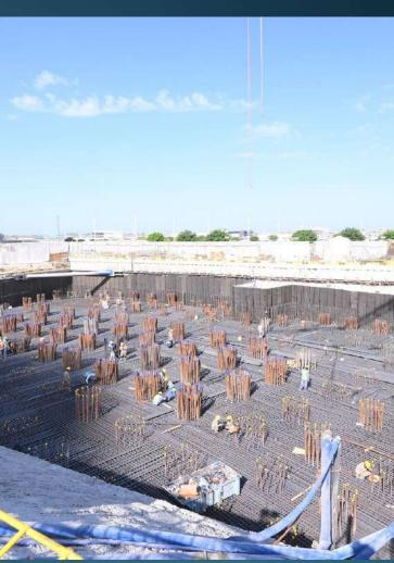
Pile breaking & substructure blockwork are in progress in Tower A. Anchoring is in progress in Tower B. Pile breaking & blinding works are in progress in Tower C.
