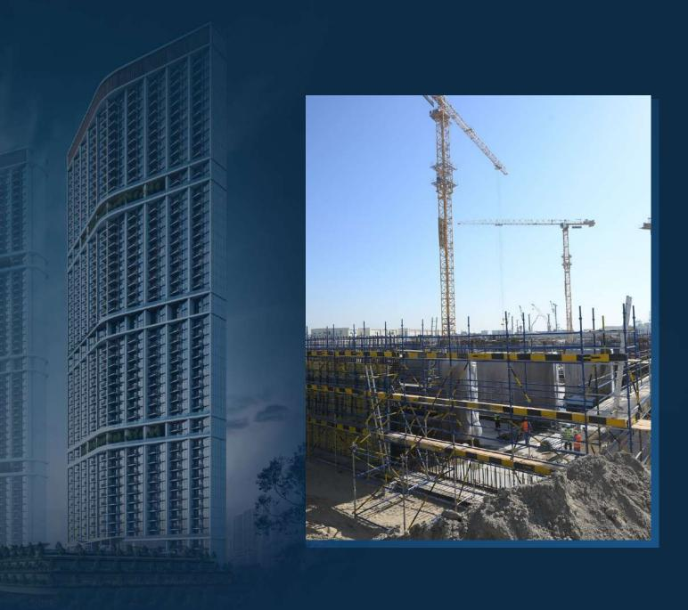
Construction of the project is proceeding favorably well. Ground floor slab and podium pile cap works are in progress. Façade works are yet to commence. Internal finishing works are yet to commence.
