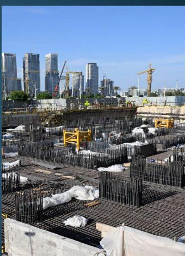
Raft works completed & verticals in progress in Tower A. Enabling works in progress at Tower B and raft works in progress a Tower C. Façade and internal finishes works are yet to commence.
