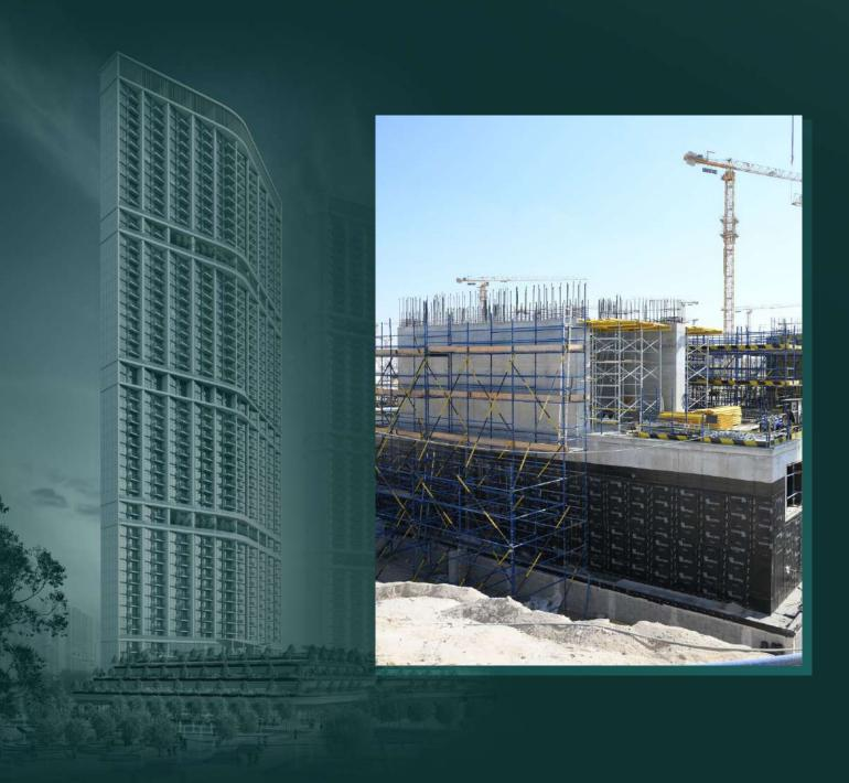
Construction of the project is proceeding favourably well. Ground floor slabs have been completed, and ACS installations are in progress. Works are yet to commence for the façade and for internal finishes.
