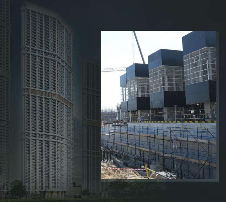
Construction of the project is proceeding favourably well. GF to L1 verticals and ACS installations have been completed with L1 to L2 verticals are in progress. Works are yet to commence for the façade and for internal finishes.
