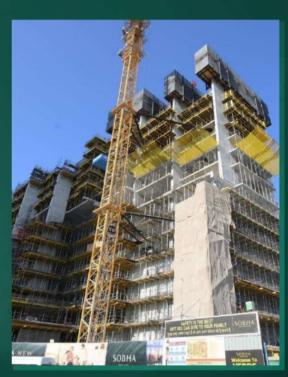
Construction of the project is proceeding favourably well. The Level 14 slab works in progress. Façade & Internal finishes work are yet to commence.
